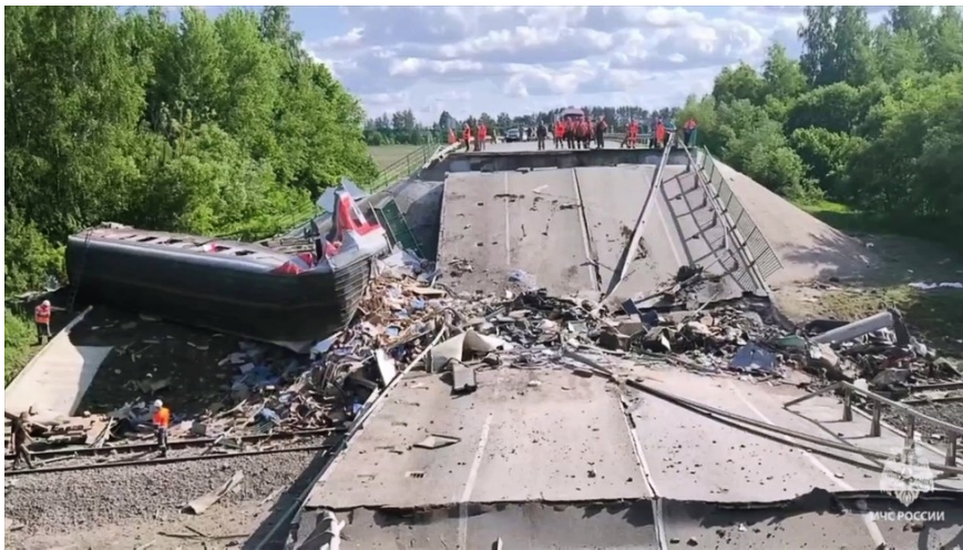
A train derailed due to a collapse of a bridge in Russia's Bryansk region. © Sputnik / Russian Emergency Situations Ministry
